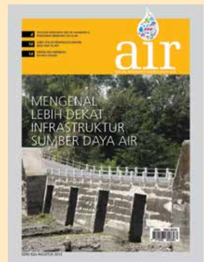
Sabo Dam Kali kuning, Yogyakarta
